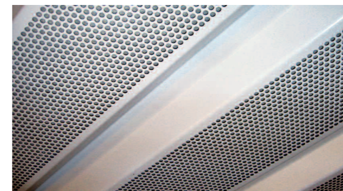
Circular perforations within the trough of the liner profile only, providing an open area of 22%.
